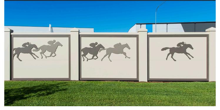
As part of a \$25M upgrade project, Warwick Farm Racecourse required a perimeter wall with an aesthetic elegance that honoured the heritage, history and tradition of the area. Additionally, the solution needed acoustic properties to shield the horses from the traffic noise caused by Governor Macquarie Drive.
